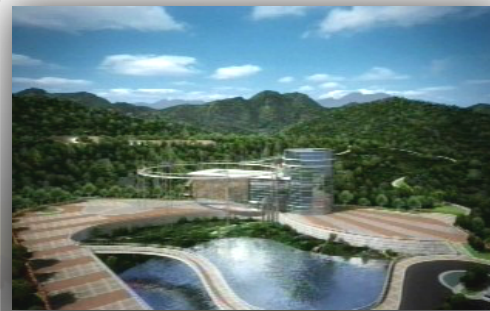
Low and Intermediate Level Radioactive Waste Disposal Facility (Under construction)
